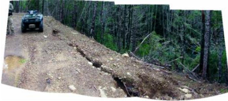
**A failing, poorly engineered and un-permitted road threatens a huge salmon-bearing stream just downslope. This road led to the clearing pictured above.**
